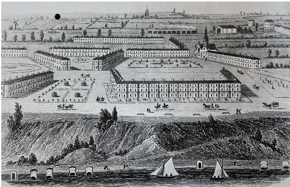
An C19 etching of the newly built Cliff Town estate and its relationship to the unmade Cliffs, with the exception of the diagonal footpath cut into the slope (Essex Record Office)
