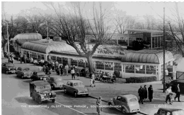
A 1956 photograph of the bandstand shelters with a horizontally glazed and curved design, typical of the 1930s. Here the earlier decorative 'Cake Stand' bandstand has been replaced with a more prosaic rectangular stage
