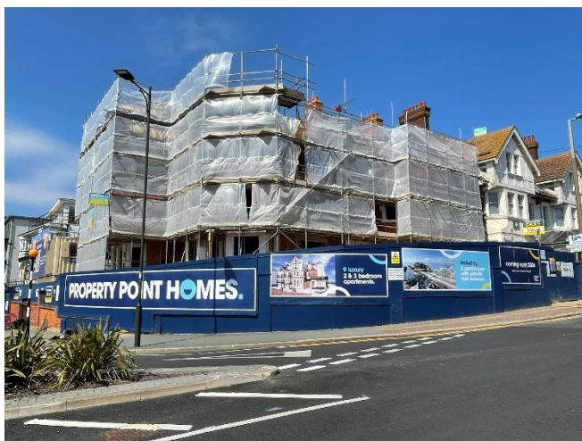
The former Beecroft Gallery site under restoration today
